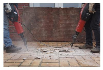
Figure 9.6: Two workers jackhammering a hard floor
